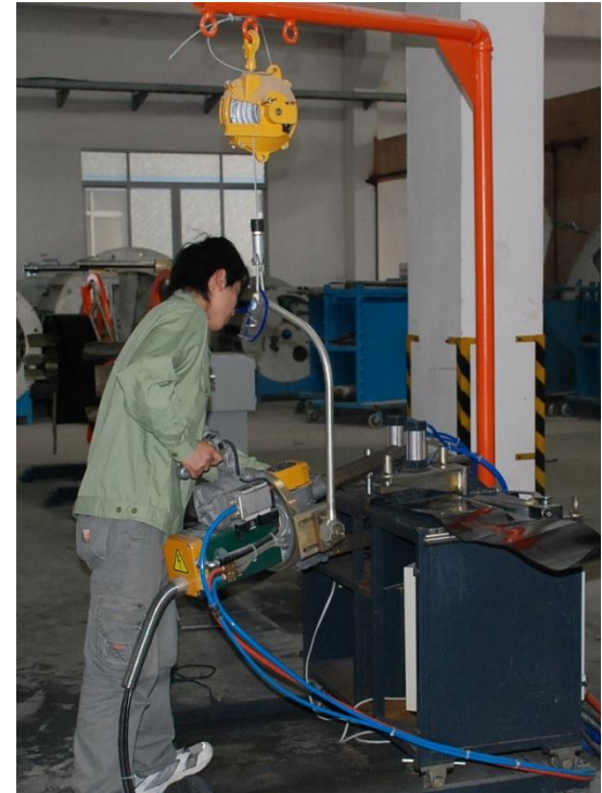
Steel sheet welding-02
